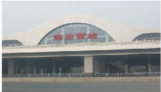
Shanxi Linfen High Speed Rail Station
