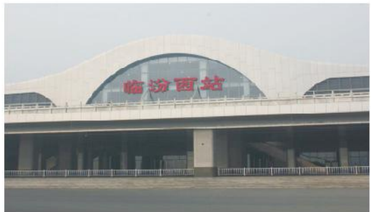
Shanxi Linfen High Speed Rail Station
